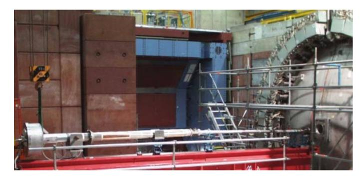
The superconducting magnet GO and the central beam pipe are prepared for installation in the liquid argon cryostat. The GO magnet provides vertical focusing and an 8 mrad bend for the electron beam in a compact coil design. The central 1 m section of the beam pipe is made from a beryllium-aluminium alloy with an elliptical cross section of  $60 \times 123$  mm and a wall thickness of 2 mm (1%  $X_0$ ).
