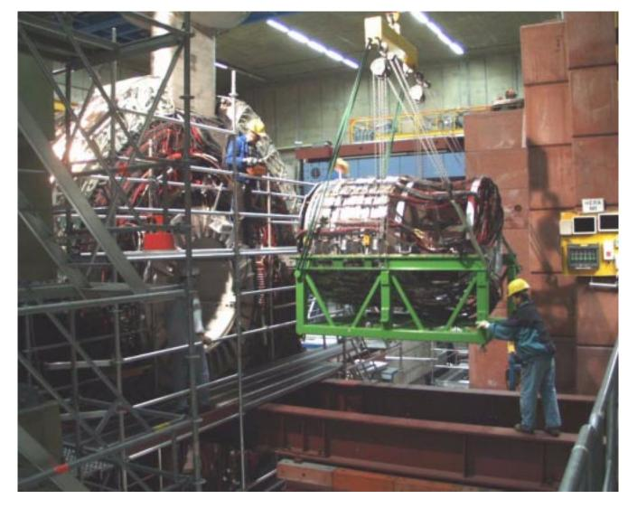
The upgraded Forward Track Detector (FTD) is being craned into position for installation. Five new and nine re-used planar drift chamber provide up to 76 measured points in 5 projections for tracks in the forward direction.
